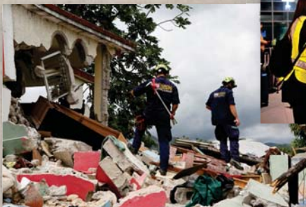
USAID DART members from Fairfax County, Virginia, survey rubble after the 2010 Haitian earthquake. Similar teams responded to natural and humanitarian disasters in South Sudan, Ethiopia, Nepal, Ukraine, and Turkey.
