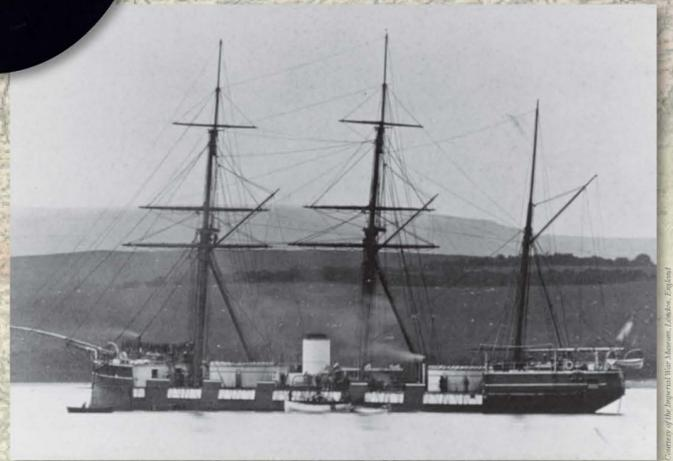
The *Wivern* was one of two ironclads built for the Confederacy by the Laird Company in Great Britain but was never delivered because of U.S. diplomatic protests. The working plans for the Laird ships included twin gun turrets, 4.5 inch-thick iron plating, and a bow reinforced with wrought iron for ramming enemy ships.
